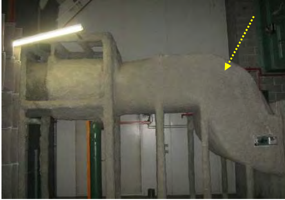
Photograph 11. Level 32: Plant room; Electrical service risers; Connecting cable trays and H.V Bus-bars - Wall and floor penetrations with fire-rated pillows (SMF insulation)
