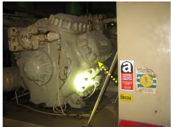
Photograph 6. Level 32: Plant room No.12; Cooling Tower section, C.W pump motors P1 to P5 - Vulcanised or 'Klingsil' gaskets between pipe sections.
